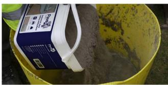
Pour the contents of the tub into the bucket. Use no more than 2 tubs at once.
