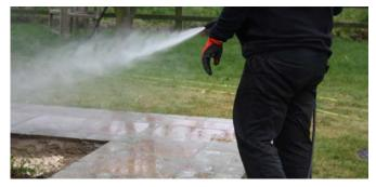
Ensure the paved area is kept completely wet throughout, until the entire area has been jointed and the joints have set firm. We suggest you mist the water on to the surface using a low pressure jet wash, pointing the lance along or upwards from the paving, never directly onto it.
