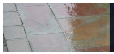
**IMPORTANT**: Washing the area too early before the Jointing Mortar has not firmed up and over watering the area can lead to discolouration. Ensure that all the residue is off the surface as once set this will be difficult to remove and may stain. Extra care should be taken when the temperature is higher as the working time will reduce.
