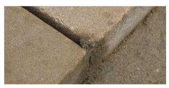
Blank off any open ended joints with modelling clay, or a firm mortar or sand.
