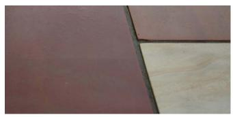
Repeat the last step until the water that runs off the surface of the paving is completely clean and clear – indicating that there is no mortar residue remaining on the surface of the paved area.
