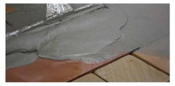
Ensure the joints are completely filled.
