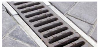
Cover any drains to prevent any mortar from getting into them, you can use plastic bags and duct tape.
