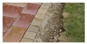
Plan the direction that you wish to brush off the excess mortar and ensure it has somewhere safe and practical to go – as any residue will set hard, could stain and cause problems if it goes into drains or similar.
