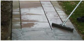
Using the rubber squeegee remove as much mortar as possible from the paved surface, whilst ensuring that all joints remain filled. Don't let the residue on the surface go matt, keep the area moist.
