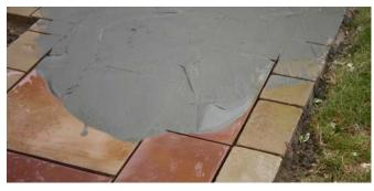
Pour the Jointing Mortar onto the pre-soaked paved area. Using a squeegee, work the slurry into the joints.
